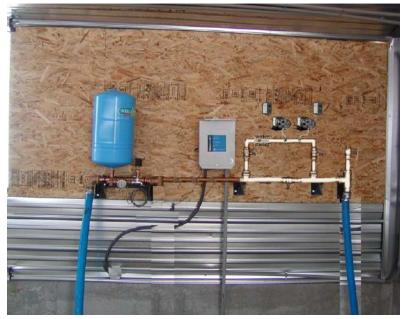
The illustration on the right shows added plumbing so that a medicator pump can be added to the water line.
